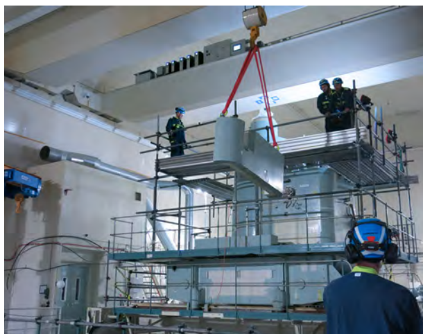
Nedmontering. Foto: Rodrigo Prieto
